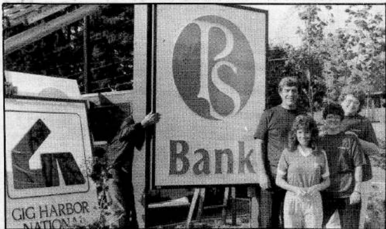
Signs of the changing times ....Don, Katherine, Cassy and Leatha are now "wearing the colors" of Puget Sound National Bank, as workmen remove the Gig Harbor National Bank sign and put up the new PSNB sign in the bank's location in uptown Key Center. KP NEWS staff photo.
