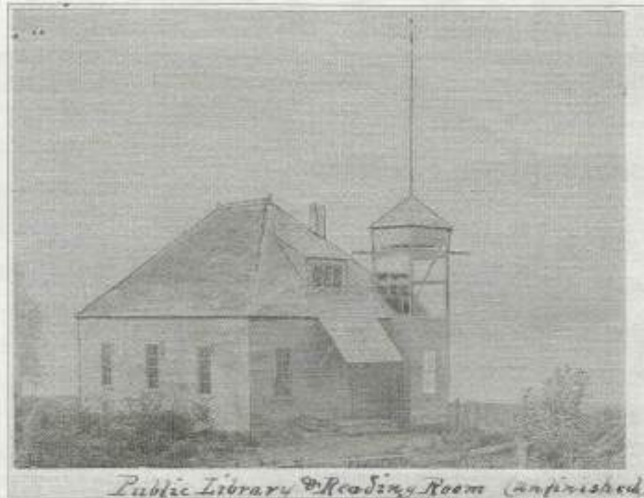
The Vaughn Library at the end of Hall Road near the bay, circa 1893.
