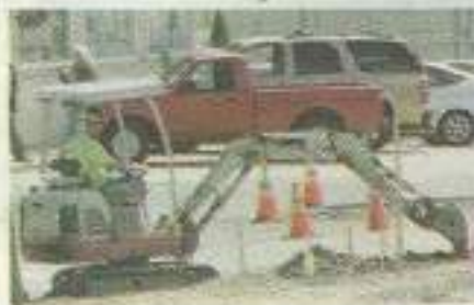
Key Center construction
